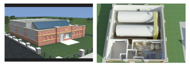
Approximately 70% of the floor space is filled with two large, insulated water tanks, each 12' diameter and 10' tall. The water temperatures within these tanks are "stratified", that is tank 1 holds the warmest water, and tank 2 the coolest. This allows the system controls to pull just the right temperature water that is needed, or to return heated water to the best location.
